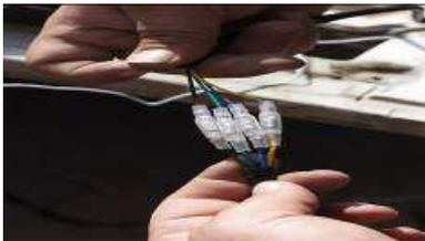
Once you have all the wires through you can connect them to each other by matching up the colors. The white wire will be wired into the taillight so make sure this is coming out the bottom of the tailgate.
