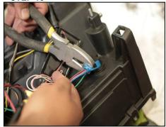
The red and blue wires will splice to the center brown wire on the parking/turn signal socket.
